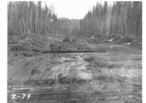
"Corduroy" paving (foreground) and a wooden culvert to deal with excessive water. [U.S. Army Corps of Engineers]
