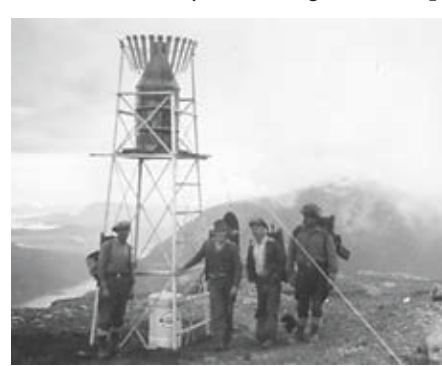
The installation of a rain gauge on Gastineau Peak near Juneau in 1941. [NOAA]
